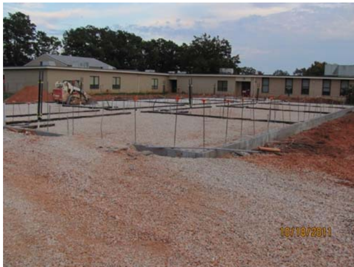
Slab Preparation for New Classrooms
